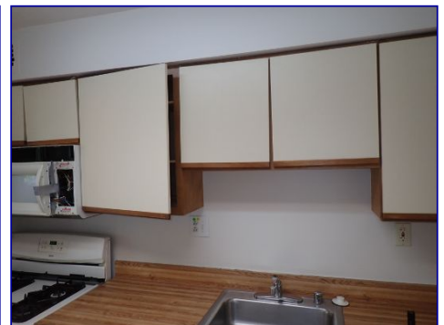
Hinges loose. Doors and drawers misaligned. Kitchen.
