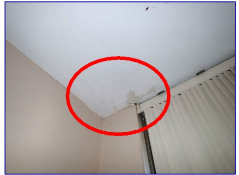
Paint failed. Rear bedroom rear corner.
