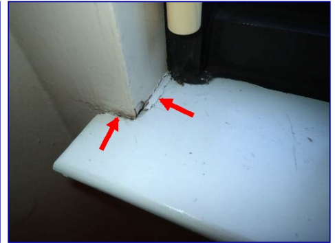
Caulk failed. Window sills.
