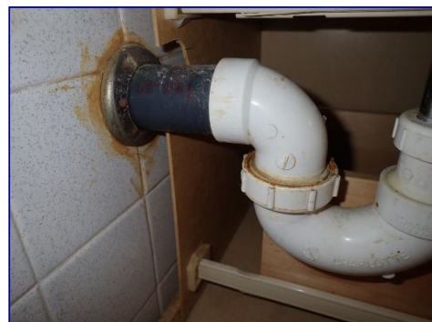
Dissimilar plastics. Water stains. Hall bathroom.
