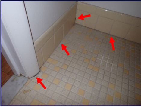
Caulk missing. Floor perimeter. Half bathroom.
