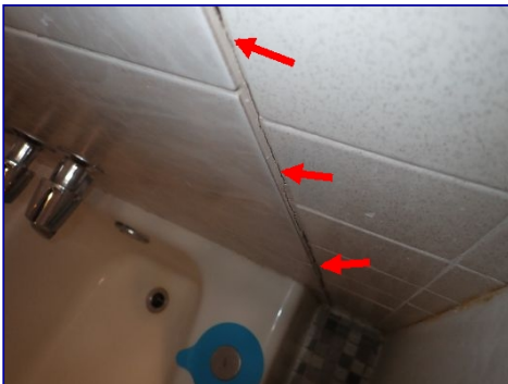
Caulk missing. Hall bathroom.
