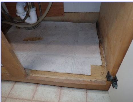
Shelf damaged. Evidence of leak. Under kitchen sink.
