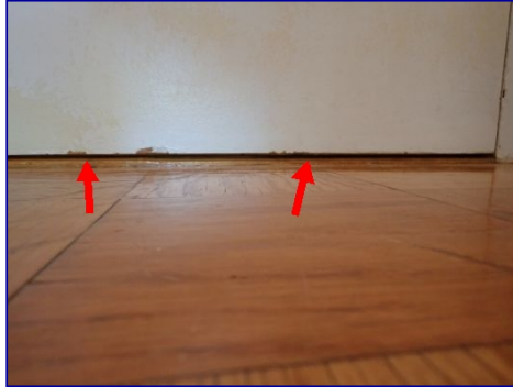
Weatherstripping missing. Entry door bottom.
