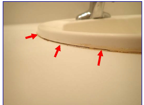
Caulk failed. Half bathroom.
