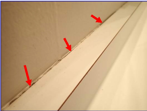
Caulk failed. Half bathroom.
