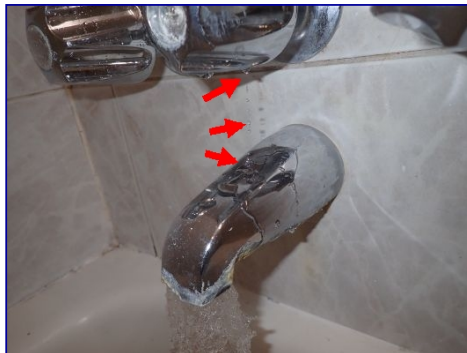
Leak visible. Diverter handle.
