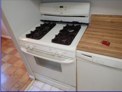
Anti-tip bracket missing.
