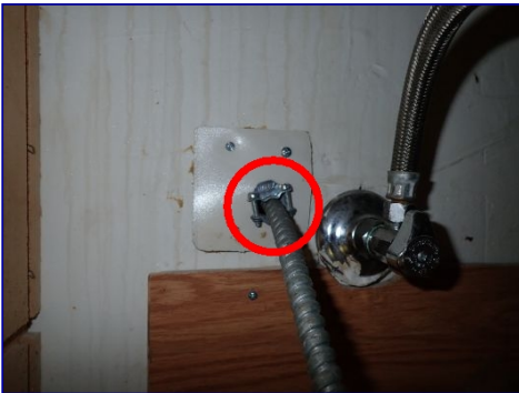
Wire clamp loose. Garbage disposal. Under kitchen sink.
