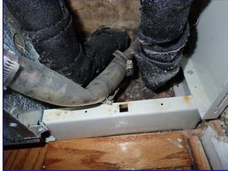
Drain pan not visible. Rear bedroom.
