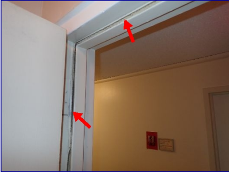
Weatherstripping missing. Entry door frame.
