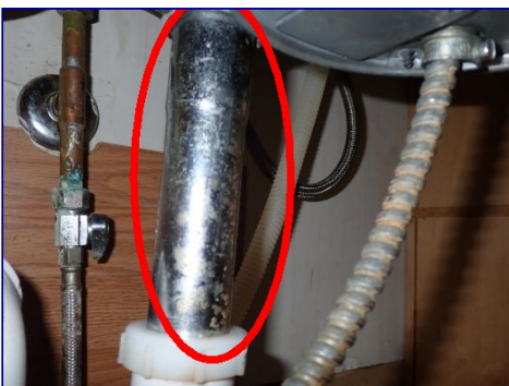
Corrosion visible. Kitchen sink tailpiece.
