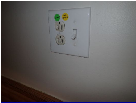
GFCI protection missing. Receptacle worn. Kitchen countertop.
