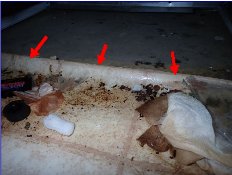
Flooring loose. Under oven.
