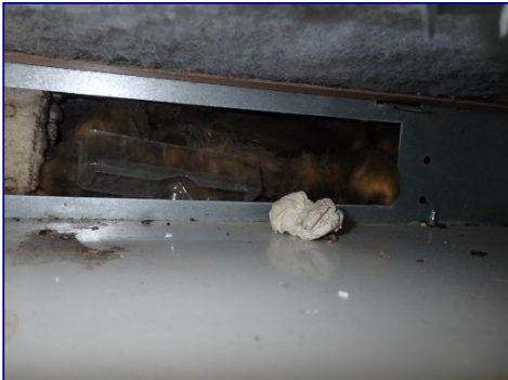
Hole in wall. Behind convector. Rear bedroom.
