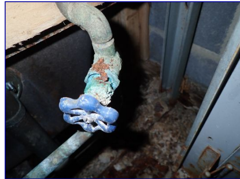
Corrosion visible. Shower shutoff valve.
