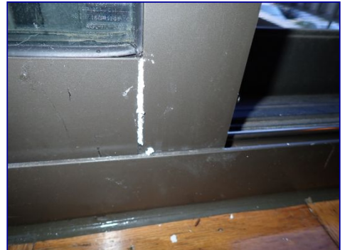
Caulk missing? Exposed insulation. Sliding door.
