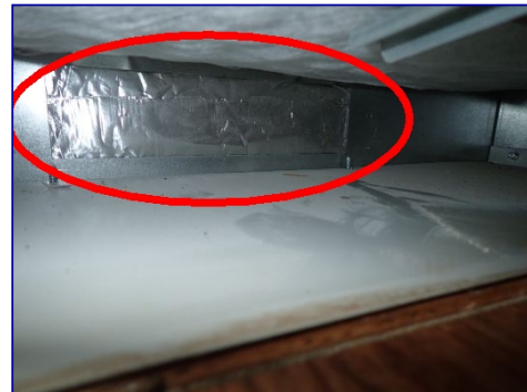
Repair visible. Tape over hole. Side bedroom.
