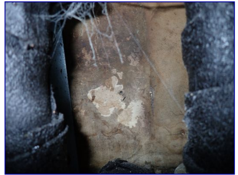
Organic growth visible. Wall behind convector. Rear bedroom.
