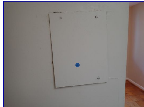
Cover loose. Phone box on kitchen wall.
