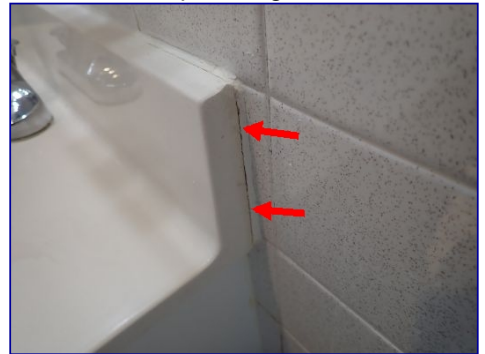
Caulk failed. Hall bathroom.
