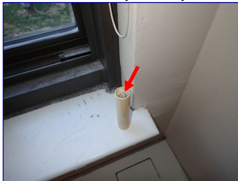
Blinds damaged. Roller wheel missing. Rear bedroom.
