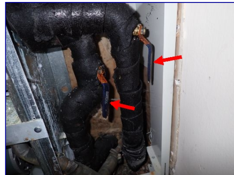
FYI: Convactor heating system supply and return water shutoff valves.
