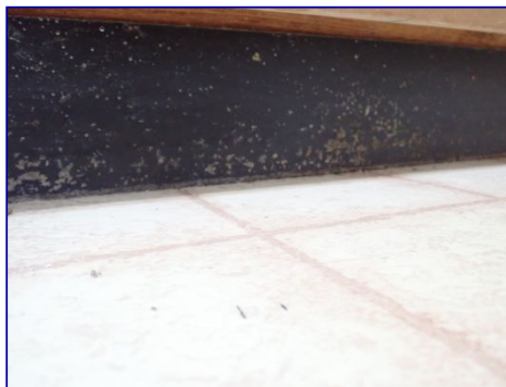
Trim damaged. Kitchen base plates.
