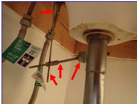
Rust and corrosion visible. Half bathroom drain stopper.
