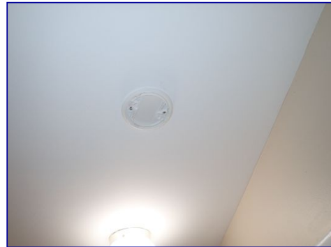
Smoke alarm missing in hall.
