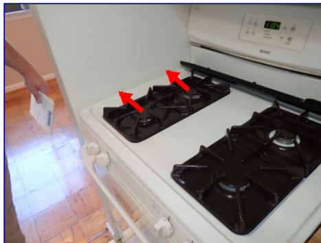
Clearance to combustibles missing.
