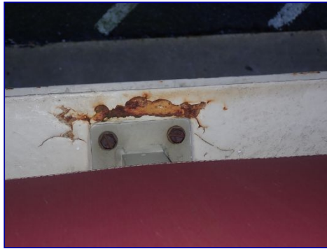
Rust visible. Paint failed. Railing post base.
