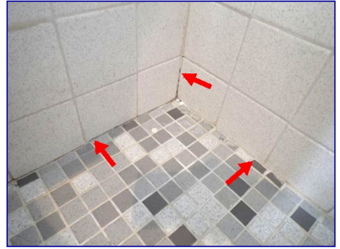
Caulk missing. Floor perimeter. Hall bathroom.
