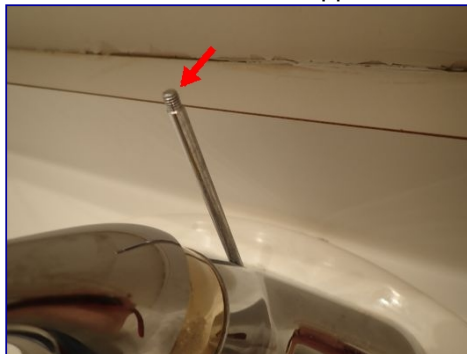
Drain stopper damaged. Knob missing. Half bathroom.
