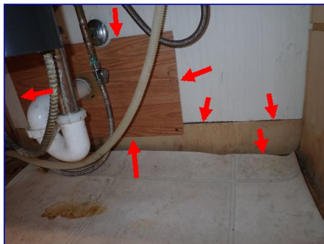
Holes in wall. Under kitchen sink.
