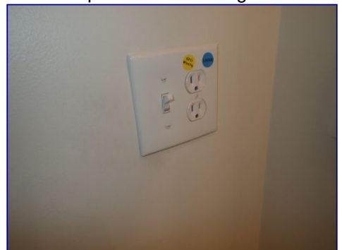
GFCI protection missing. Receptacle loose.
