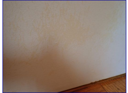
Paint failed. Entry door.
