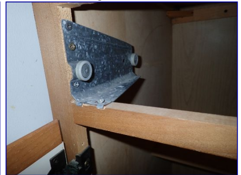
Drawer guide loose. Kitchen at refrigerator.
