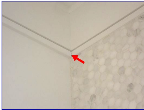
Caulk missing. Pantry.
