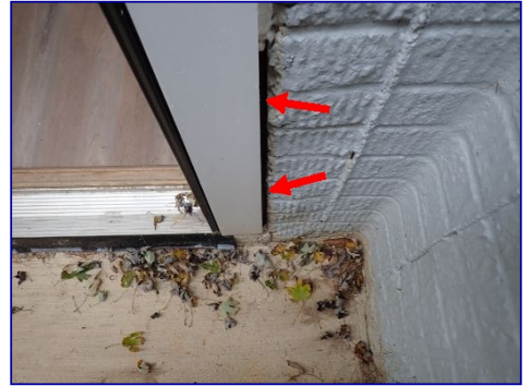
Caulk missing. Basement door frame.
