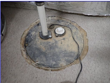
Seal missing on well cover. Utility room.
