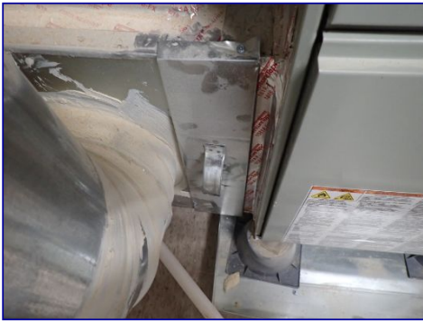
Air filter cover seal missing. Utility room.
