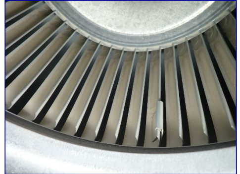
Construction dust in air handler. Loft HVAC closet.
