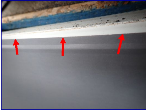
Drip edge flashing behind gutter.
