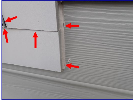
Caulk missing. Window frames.
