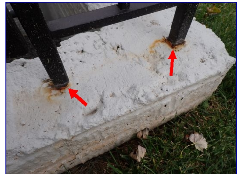
Rust visible. South side.
