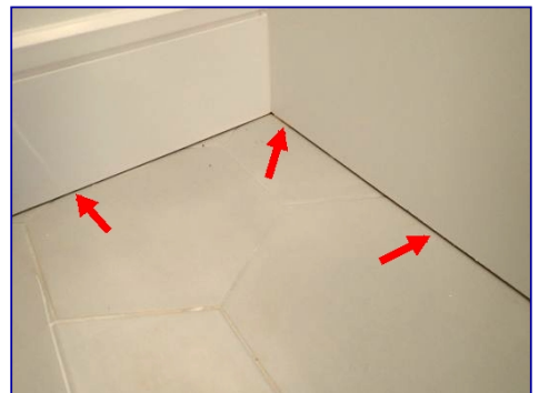
Caulk missing. Floor perimeter. Front bedroom bathroom.
