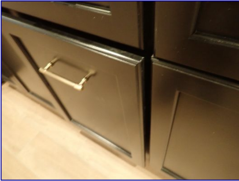
Soft-close inoperable. Basement bar.
