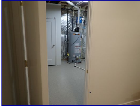
Combustion air vents not visible. Utility room.
