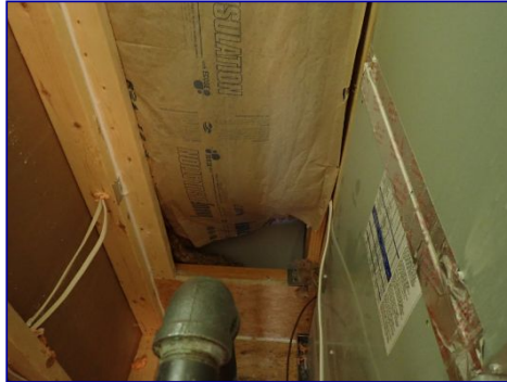
Exposed flammable backing. Loft HVAC closet.
