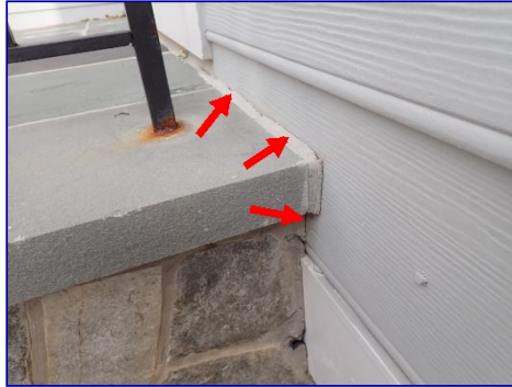
Clearance missing. Siding-to-surface. Rear.
