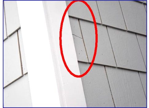
Siding damaged. Upper front side.
