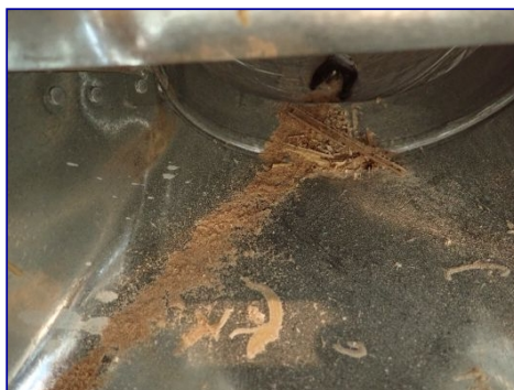
Register boxes dirty. Construction debris.
