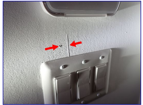
Hole in wall. Paint drips. Mudroom.
