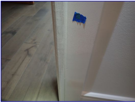
Paint flashing. Kitchen.
