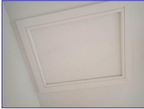
Seal missing. Ceiling hatch. Laundry room.
