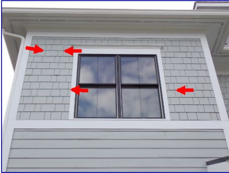
Keyways aligned. Front.
