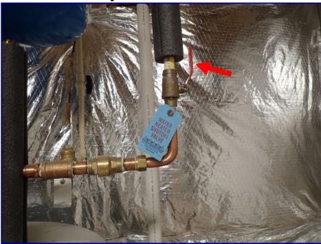
FYI: Water heater cold water shutoff valve. Utility room.
