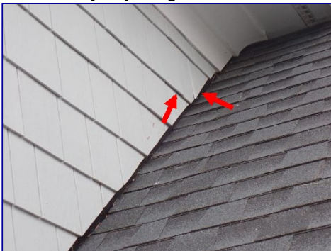
Siding loose. Upper front side.
