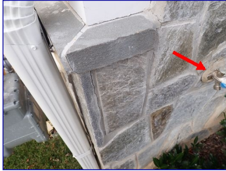
Hose bibb loose. Sealant failed. Front.
