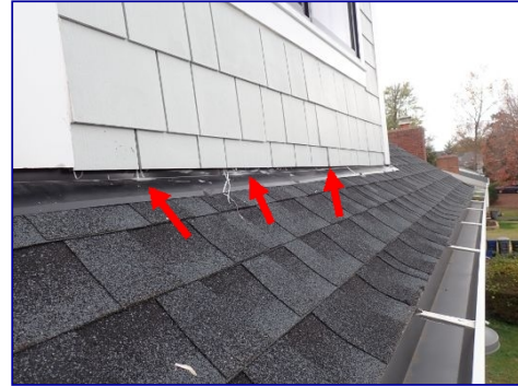
Paint on flashing. Upper front.
