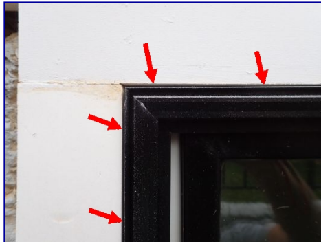
Caulk missing. Window frames.
