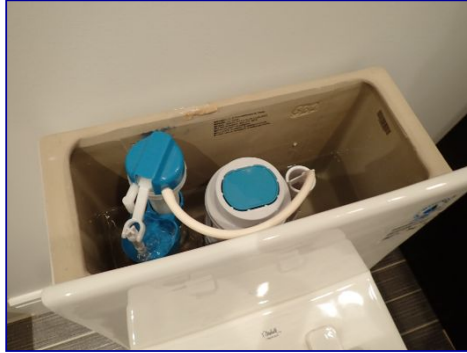
Flush out of adjustment. Basement bathroom.
