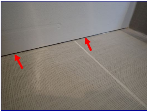
Caulk missing. Floor perimeter. South bedroom bathroom.
