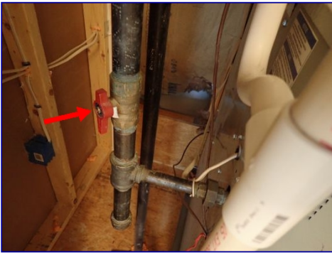
FYI: Furnace gas shutoff valve. Loft HVAC closet.
