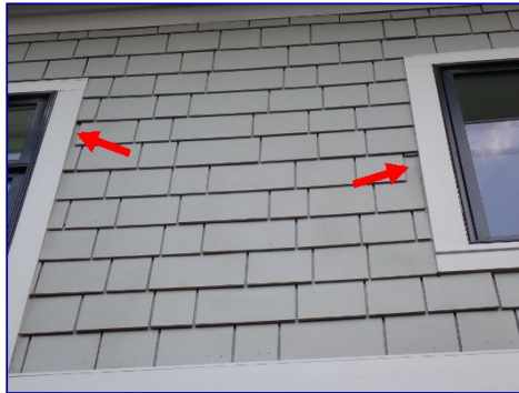
Shingle tabs missing. South side.
