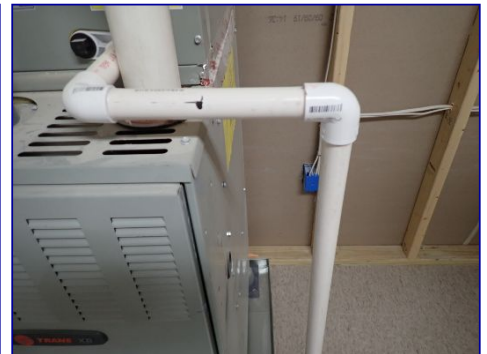
Trap missing. Condensate drain line. Utility room.
