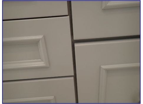
Doors and drawers misaligned. Master bathroom.
