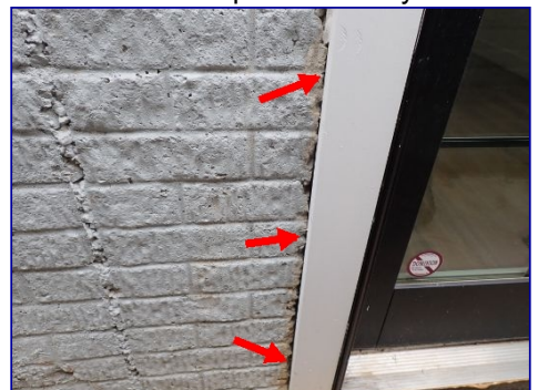
Caulk missing. Basement door frame.
