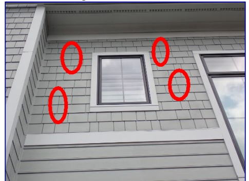
Keyways aligned. South side.
