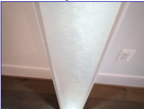
Paint flashing. Sunroom at kitchen.
