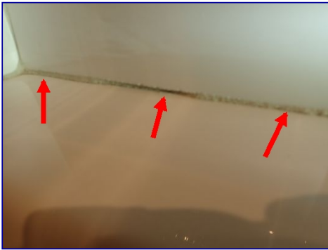
Caulk missing. Bathtub perimeter. Basement bathroom.
