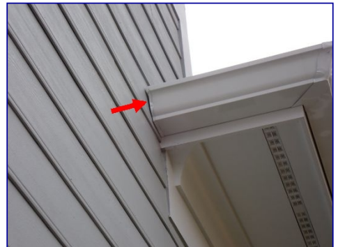
Gutter end clearance missing. Gutters at siding.
