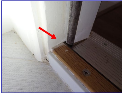
Weatherstripping missing. Corner seal. Garage entry door.
