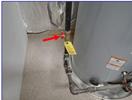
FYI: Water heater gas shutoff valve. Utility room.
