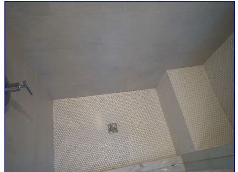
Caulk missing. North bedroom bathroom.
