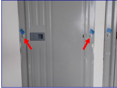
Cover screw hole stripped.
