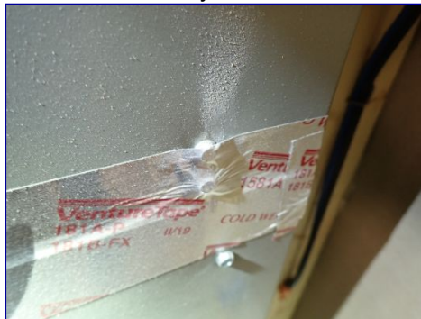
Sealant failed. HVAC tape. Utility room.
