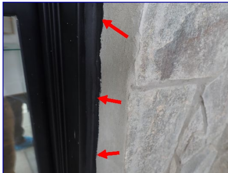
Casing bead not visible. Stone at trim.
