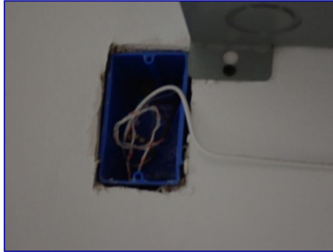
Cover plate missing. Utility room ceiling.
