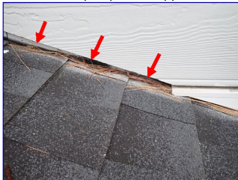
Clearance missing. Siding-to-roofing. Lower rear.
