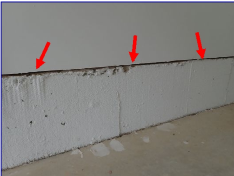
Hole in garage firewall.
