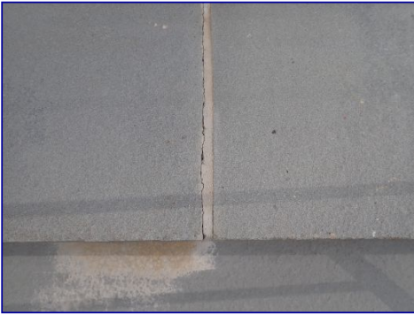
Mortar cracked. Rear.
