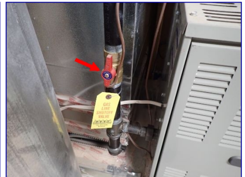
FYI: Furnace gas shutoff valve. Utility room.
