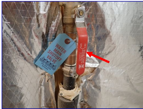
FYI: Main water shutoff valve. Utility room.
