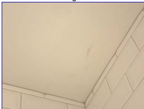
Stains on ceiling. Front bedroom bathroom.
