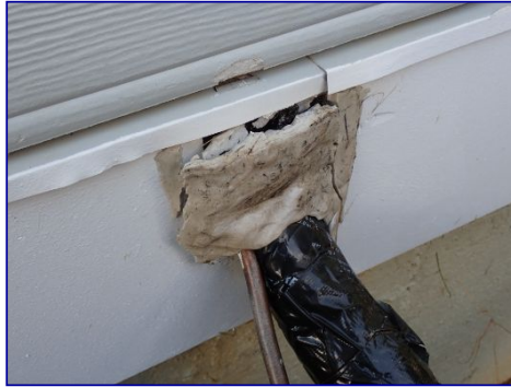
Sealant failed. North side.
