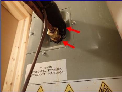
Sealant missing. Cabinet penetrations. Loft HVAC closet.
