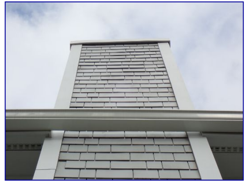
Siding loose. Chimney.
