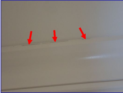
Caulk failed. Upstairs hall crown molding.
