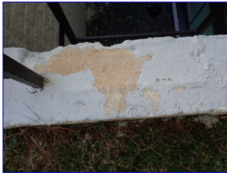
Paint failing. North side window well.
