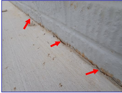
Sealant missing. Rear.
