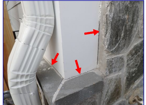
Caulk missing. Front south corner.
