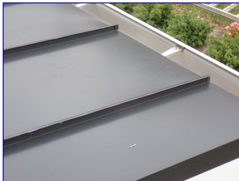
Metal standing seams single-locked. Lower front.
