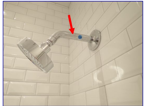
Shower mast loose. Front bedroom bathroom.
