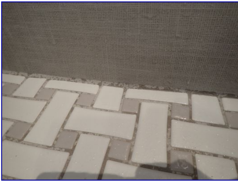
Grout sealant not visible.
