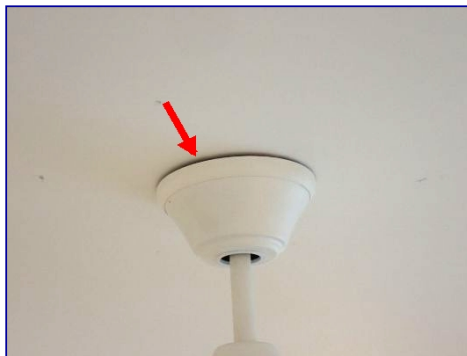
Ceiling fan mount misaligned. Loft bedroom.
