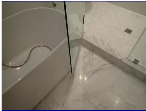
Door bumper missing. Door hits bathtub. Master bathroom.
