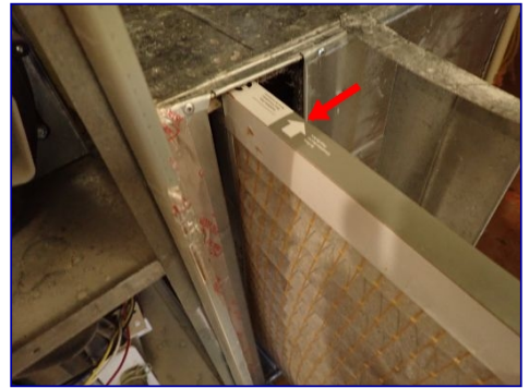
Air filter backwards. Loft HVAC closet.
