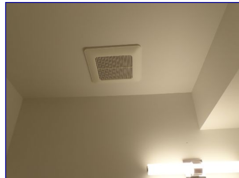
Exhaust fan inoperable? Front bedroom bathroom.
