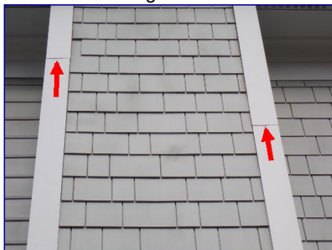
Caulk missing. Chimney.
