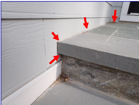
Clearance missing. Siding-to-surface. Rear.
