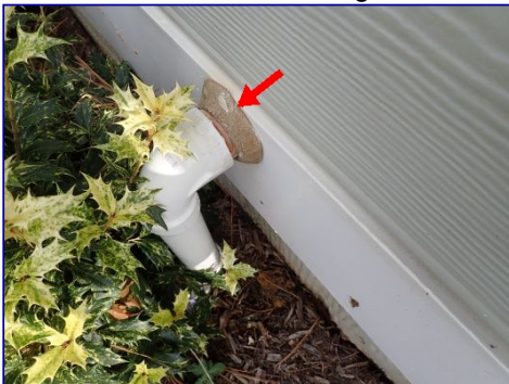
Sealant failed. Rear.
