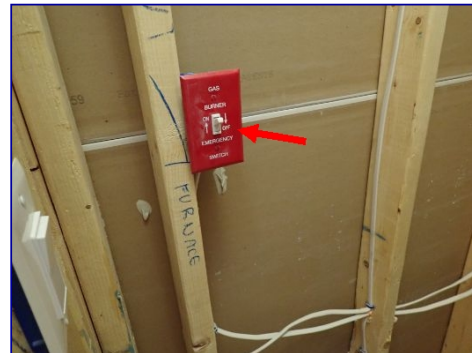
FYI: Air handler service disconnect. Loft HVAC closet.
