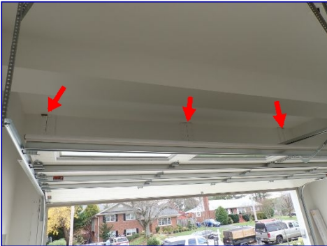
Hole in garage firewall.
