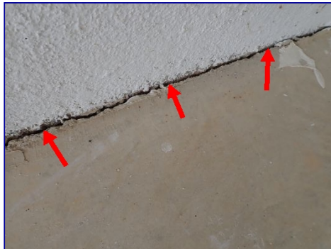
Sealant missing. Floor perimeter. Family room.
