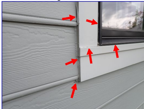
Caulk failed and missing. Window frames.
