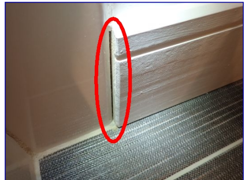
Paint missing. Caulk missing. Baseboard at bathtub. Basement bathroom.
