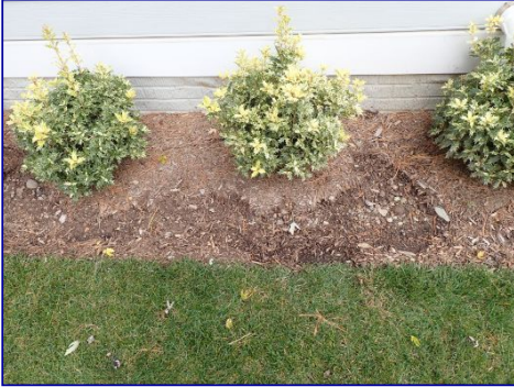
Evidence of gutter overflow. Rear.
