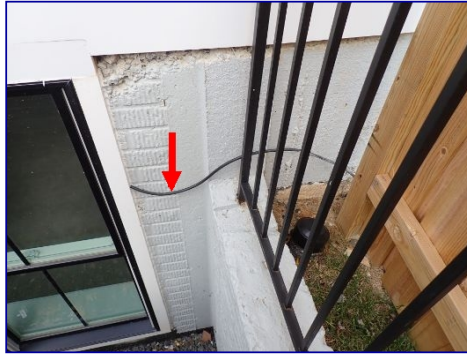
Ground wire loose. South side at meter.
