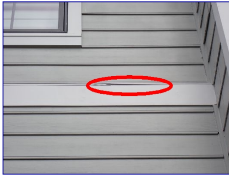
Flashing bent. South side.
