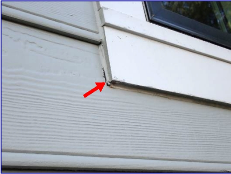
Caulk failed. North side.
