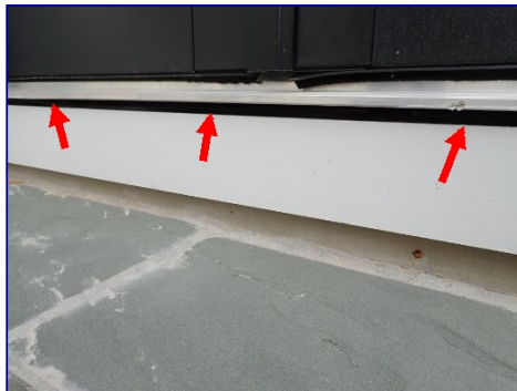
Sealant missing. Door threshold. Rear.
