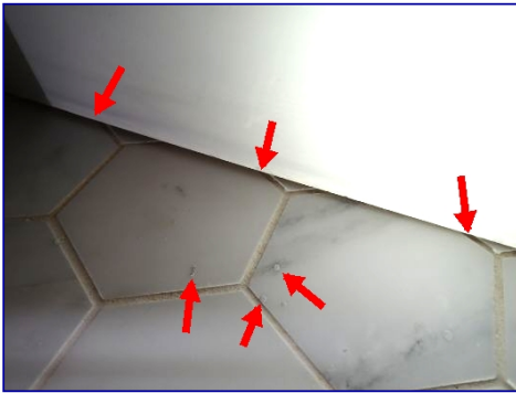
Caulk missing. Floor perimeter. Half bathroom.
