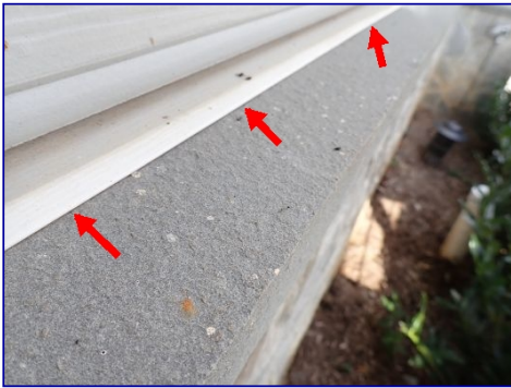
Sealant missing. Flashing at stone.
