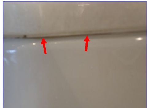
Caulk failed. Sink under countertop. v
