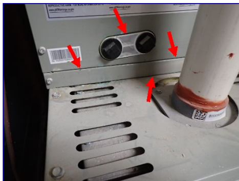
Sealant missing. Cabinet penetrations. Utility room.
