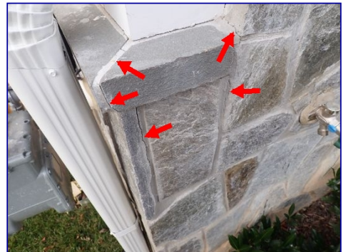
Mortar cracked. Front south corner.
