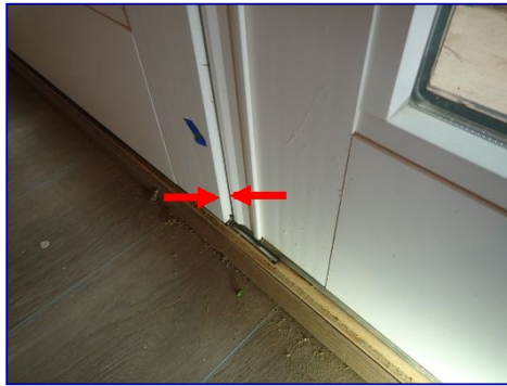
Doors misaligned. Basement.
