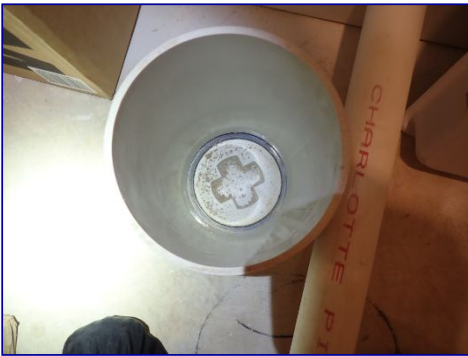
FYI: Backwater valves in media room closet and utility room.
