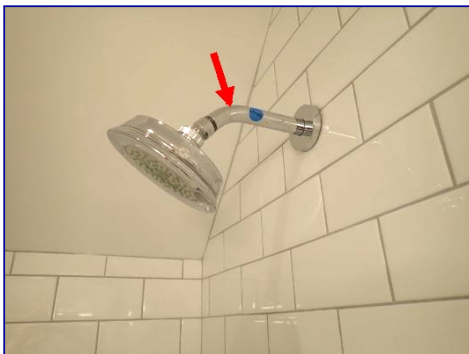
Shower mast loose. Loft bathroom.
