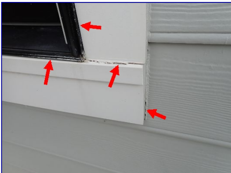
Caulk failed and missing. Rear.
