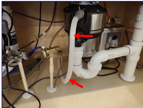
Dishwasher drain high loop missing. Under kitchen sink.
