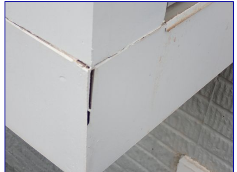
Trim warped. Chimney.
