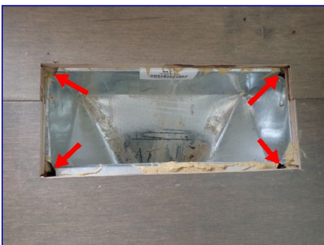
Sealant missing around floor register boxes.
