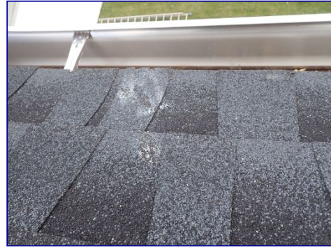
Paint on roofing. Upper front.
