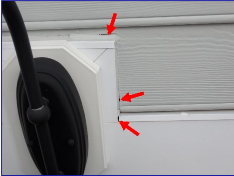
Caulk failed. South side.
