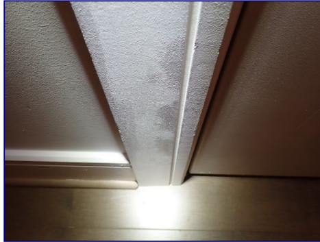
Paint flashing. Upstairs hall.
