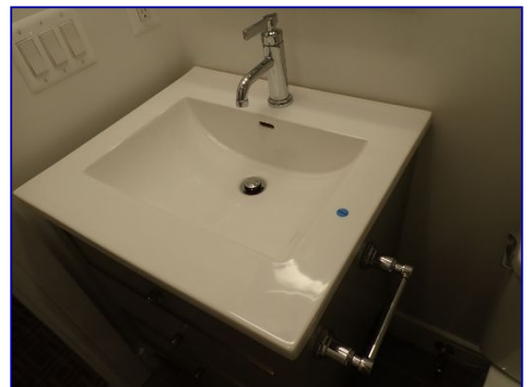
Sink loose. Loft bathroom.
