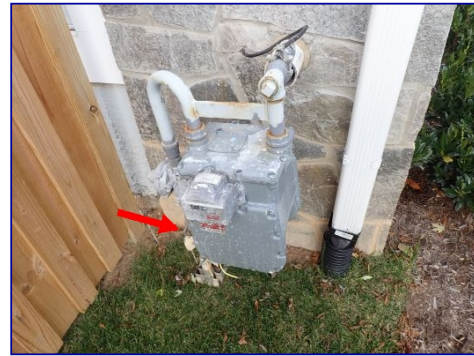
FYI: Main gas shutoff valve at meter. South side front corner.
