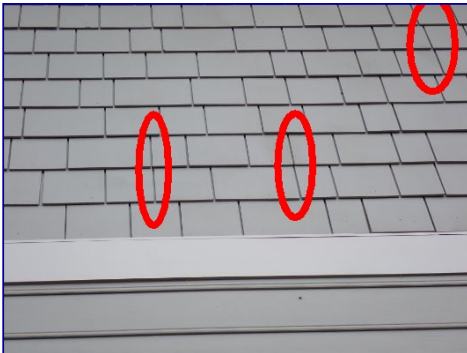
Keyways aligned. South side.
