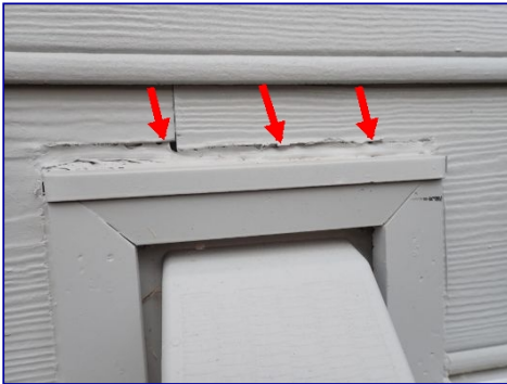
Caulk failed. South side.
