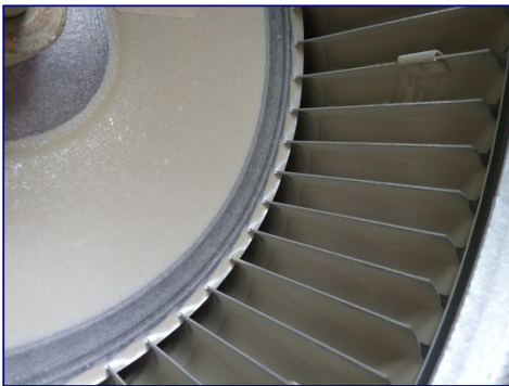
Construction dust in air handler. Utility room.
