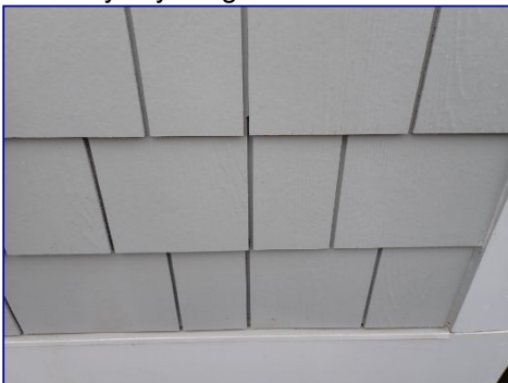
Keyways aligned. South side.
