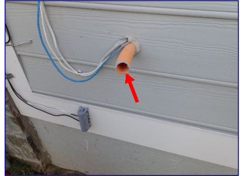
Sealant missing on conduit. North side.
