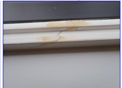
Window frame damaged. Paint missing. Family room.
