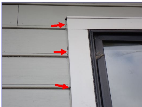
Caulk failed. North side.
