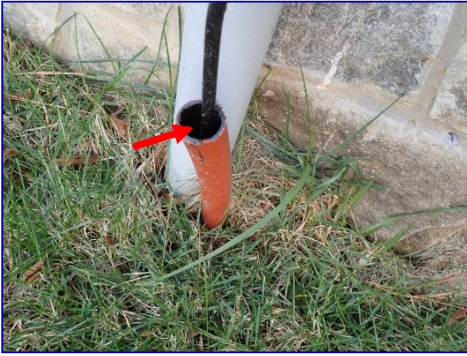
Sealant missing on conduit. North side.
