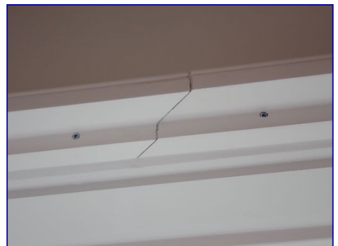
Filler missing. Master bedroom shutters.
