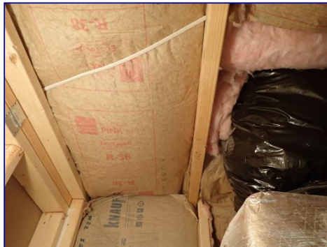
Exposed flammable backing. Loft HVAC closet.
