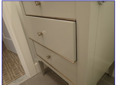
Soft-close inoperable. Loft bathroom.
