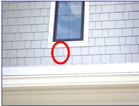
Siding damaged. Front.
