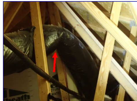
Duct bend excessive. Attic.
