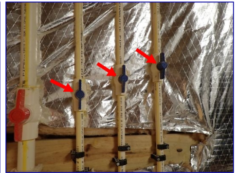
FYI: Exterior hose bibb shutoff valves. Utility room.
