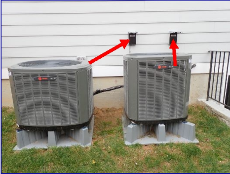
FYI: A/C service disconnect. North side.
