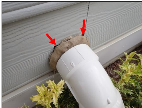
Sealant failed. Rear.
