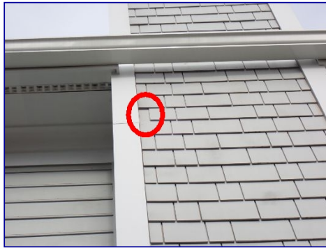
Shingle tab missing. Chimney.
