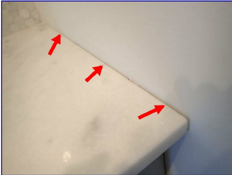
Caulk missing. Pantry.
