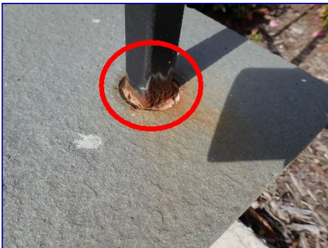
Anchoring cement low. Rust visible. Front.
