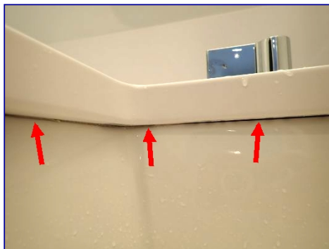
Caulk not visible. Sink under countertop. Bathrooms.
