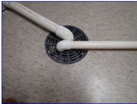
Pipes drain on cover. Utility room.
