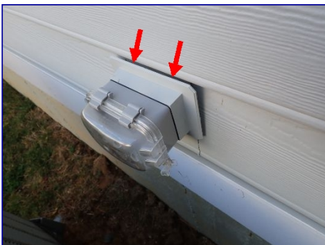
Sealant missing. North side.
