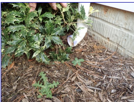
Sump pump extension missing. Rear.
