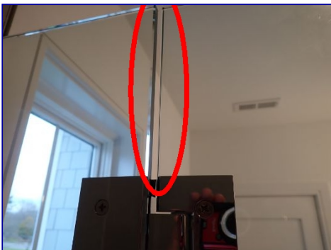
Seal missing on shower door. South bedroom bathroom.
