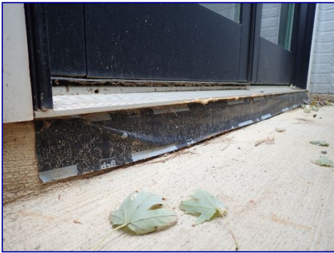
Trim missing. Under basement door threshold.
