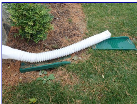
Downspout extension negative slope. Rear north corner.
