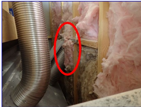
Clearance to combustibles missing. Family room.
