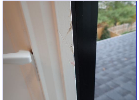
Window frame damaged. Paint missing. Master bathroom.
