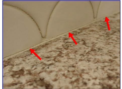
Caulk missing. Basement bar.
