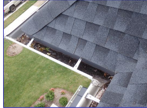
Debris in gutter. Standing water. Upper front.
