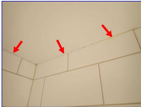
Caulk missing. Basement bathroom tile at ceiling.
