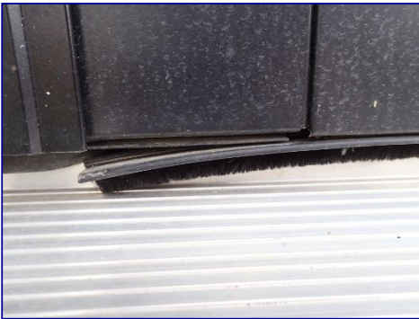
Weatherstripping loose. Rear.
