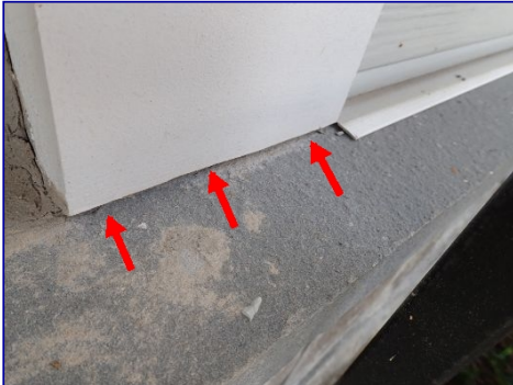
Caulk missing. Trim at stone.
