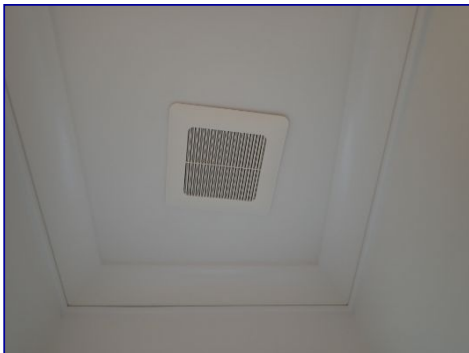
Exhaust fan misaligned. Study half bathroom.
