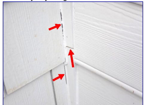
Caulk failed. Chimney.
