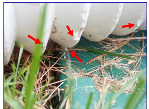
Downspout extension damaged. Rear north corner.
