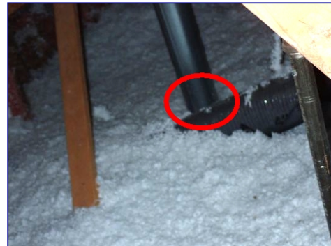
Insulation in contact with flue.
