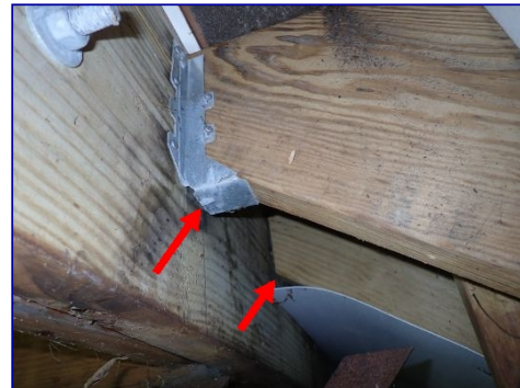
Joist hanger installed. Stair stringer connector not visible.
