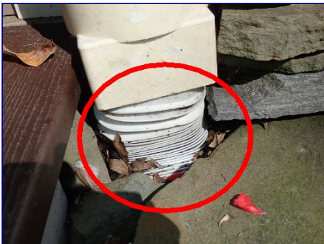
Flexible drain extension below grade. Inverted connection. Drain pipe not extended. Rear.
