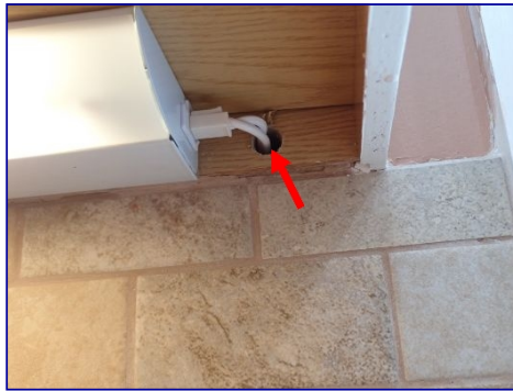
Concealed wiring. Under-cabinet countertop lights. Kitchen.
