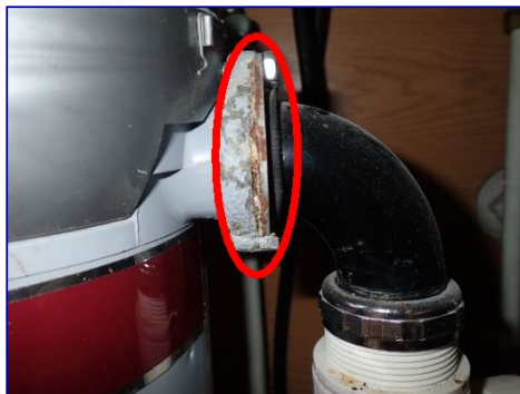
Rust and corrosion visible.
