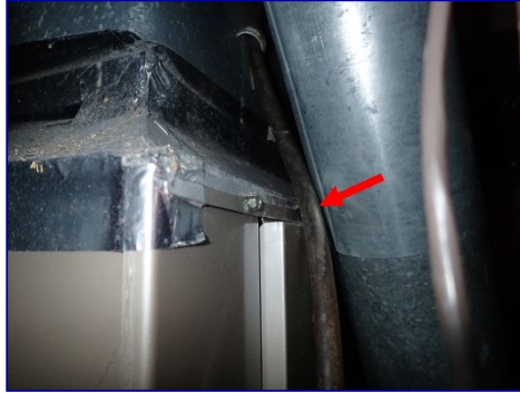
Clearance missing. Humidifier drain line. Utility closet.
