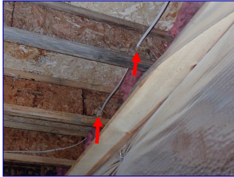
Joist hole proximity to support. Basement storage room.
