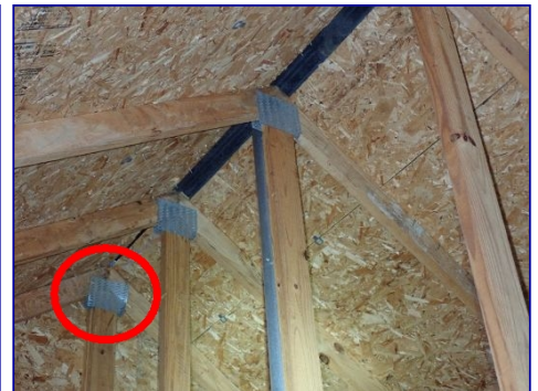
Gusset plate damaged.
