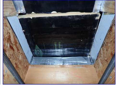
Seal missing. Pull-down stairs cover.
