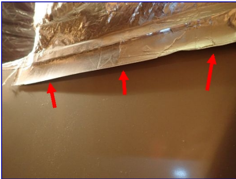
Sealant failed. HVAC tape. Attic.
