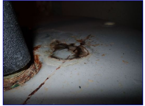
Water stain. Rust visible. Utility closet.
