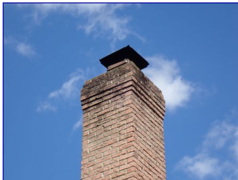
Chimney crown not visible.
