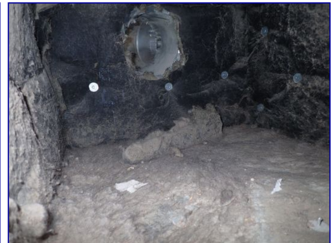
Duct dirty. Return air in utility room.
