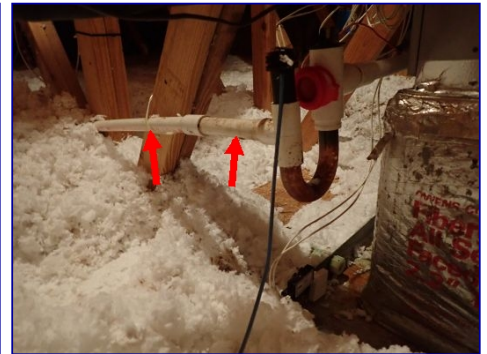
Insulation missing. Condensate drain line. Attic.
