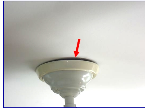
Ceiling fan mount misaligned. Green bedroom.
