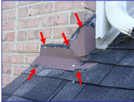
Sealant failed. Front corner.
