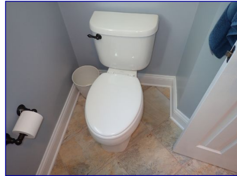
Toilet loose at floor anchor bolts. Upstairs hall bathroom.
