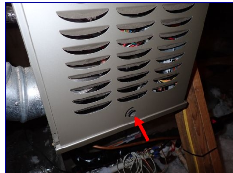
Cover loose. Clasp missing. Attic.
