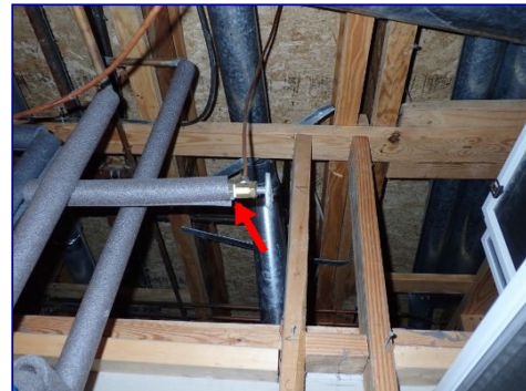
Water stains. Refrigerator water line shutoff valve. Utility closet.
