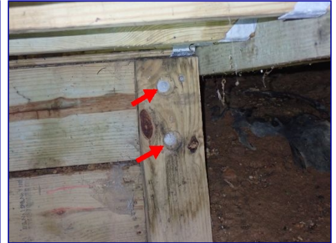
Carriage bolts installed. Washers missing.
