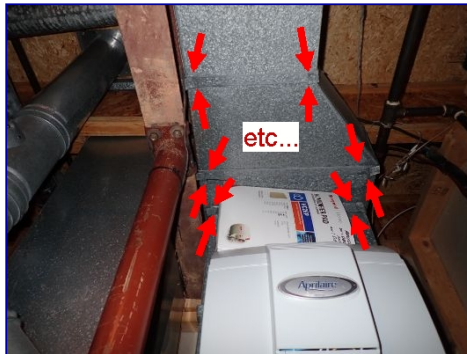
Sealant missing. Joints and seams. Utility closet.
