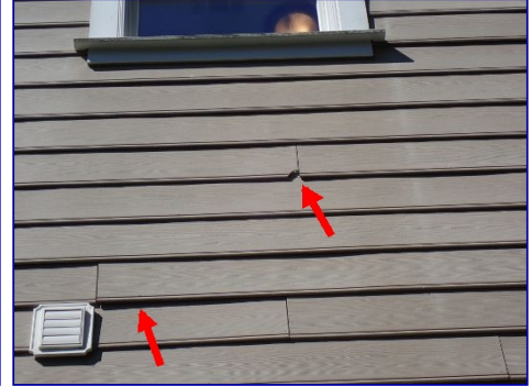
Siding loose and damaged. SE side.
