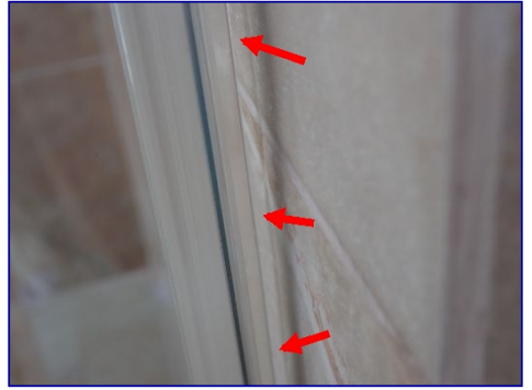
Gap in door seal. Master bathroom.
