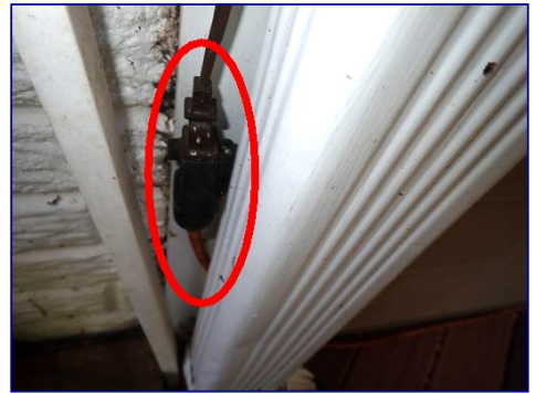
Extension cord wiring. Rear lights.
