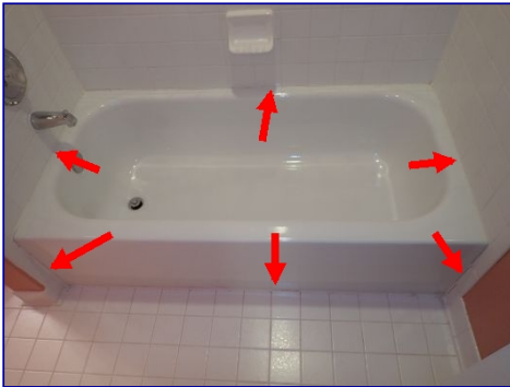
Caulk failed. Bathtub perimeter. Basement bathroom.
