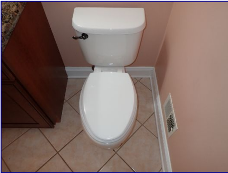
Toilet loose at floor anchor bolts. Half bathroom.
