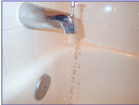
Diverter leaking. Basement bathroom.
