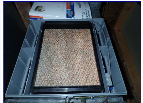
Humidifier water panel dirty. Utility closet.
