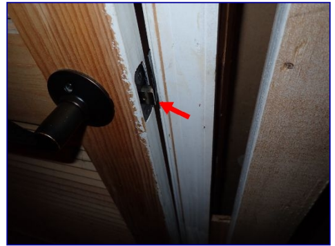
Strike plate misaligned. Utility closet.
