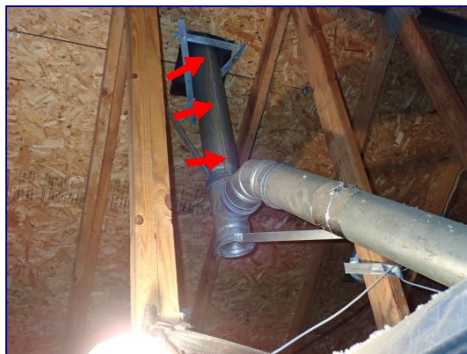
Water stain. Attic furnace flue.
