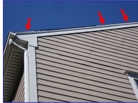
Overhang short. Roof rakes.
