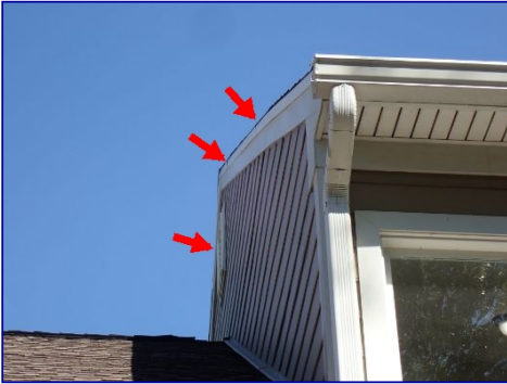
Overhang short. Roof rakes.
