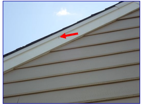
Loose nail. Garage rake.
