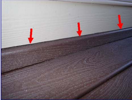
Clearance missing. Rear deck.
