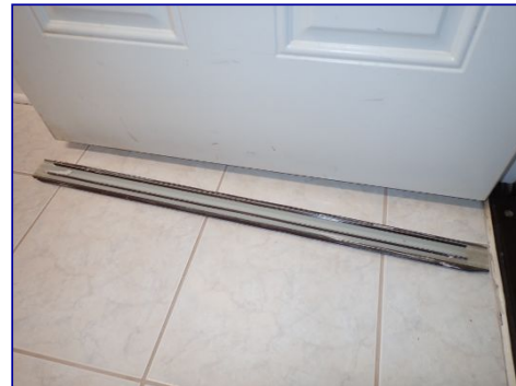
Garage entry door weatherstripping seal missing. Door bottom weatherstripping loose.
