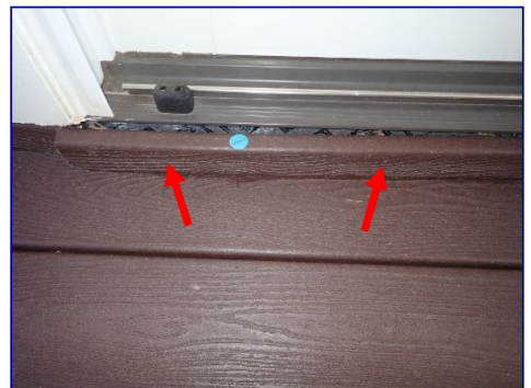
Trim loose. Under rear door threshold.
