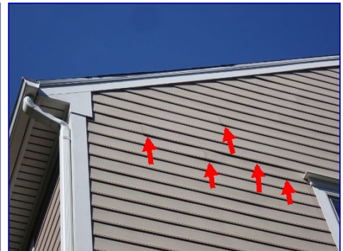
Siding loose. SE side.
