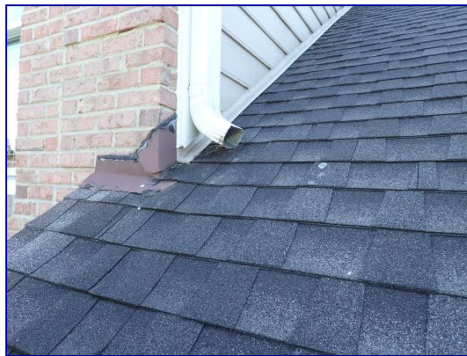
Downspout drains on roof.
