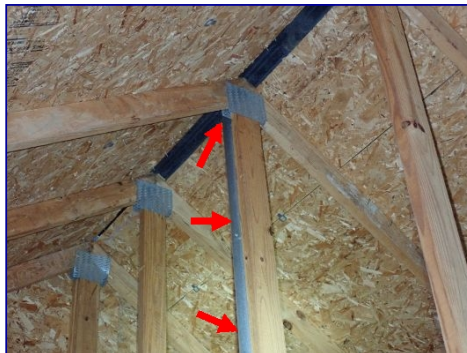
Exhaust vents to ridge vent. Insulation missing.
