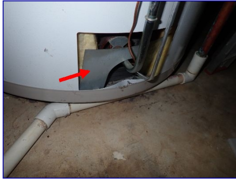
Flame shield loose.
