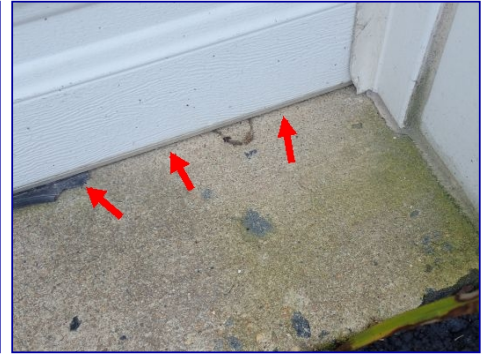
Weatherstripping damaged. Both doors.
