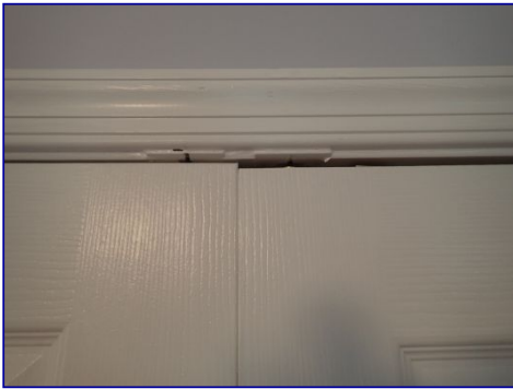
Doors misaligned. Basement bedroom closet.
