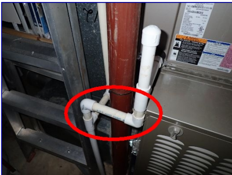
Trap missing. Condensate drain line. Utility closet.
