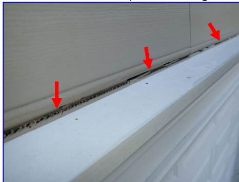
Clearance missing: siding-to-horizontal trim. Caulk failed. Garage door frame.
