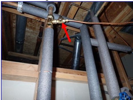
FYI: Humidifier water shutoff valve. Utility closet.
