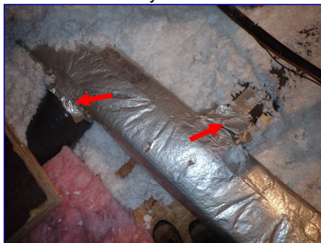
Sealant failed. HVAC tape. Attic.
