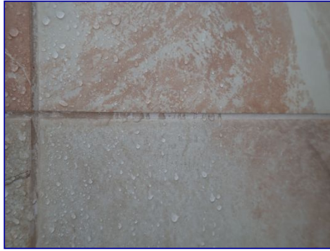
Grout sealant not visible.
