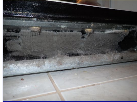
Coils dirty. Refrigerator bottom.
