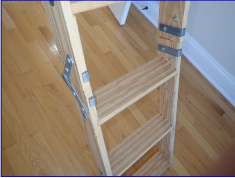
Pull-down stairs too long. Hardware loose.
