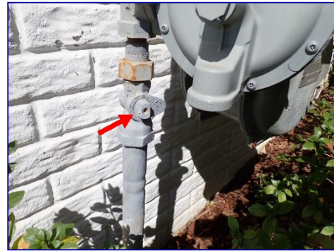
FYI: Main gas shutoff valve at meter. SE side.
