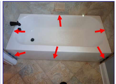
Caulk missing. Bathtub perimeter. Upstairs hall bathroom.
