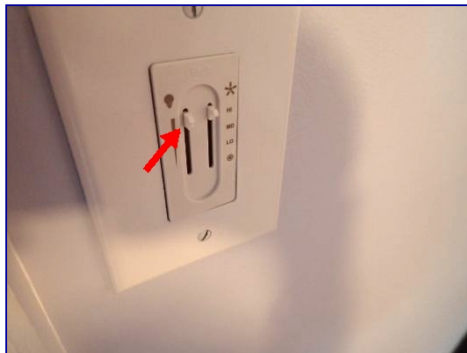
Dimmer inoperable. Basement bedroom ceiling fan.
