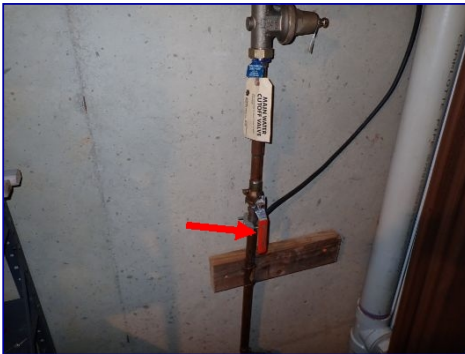
FYI: Main water shutoff valve. Basement storage room.
