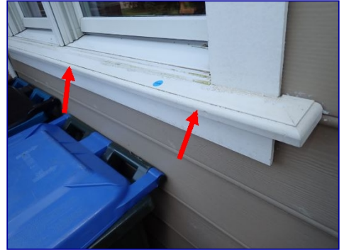
Trim loose. NW side window sill.
