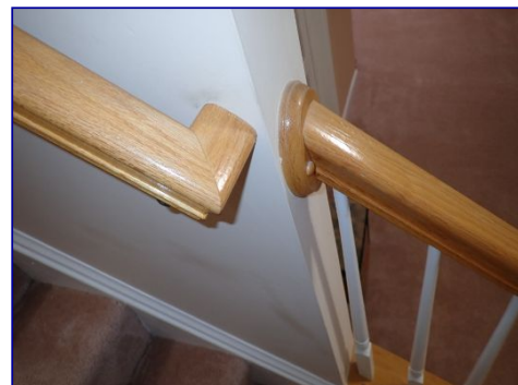
Broken transition. Basement stairwell.
