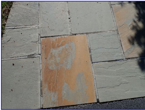
Mortar cracked. Front.
