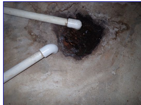
Pipe drains on floor. Pipe drains on cover. Cover rusted. Pipes loose. Utility closet.
