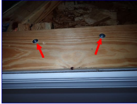
Fasteners wrong type. Pull-down stairs frame.
