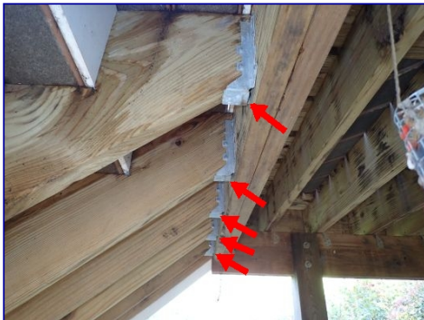
Joist hangers installed.
