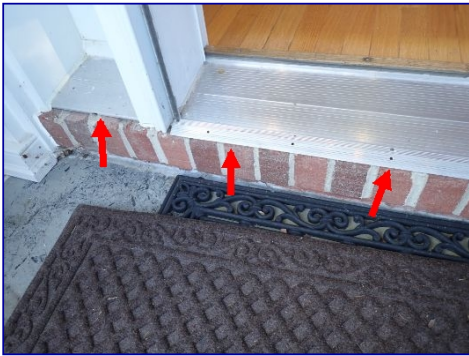
Sealant missing. Front door threshold.
