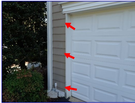
Trim missing. Garage door frame.
