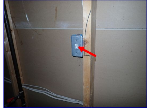
FYI: Air handler service disconnect. Utility closet.
