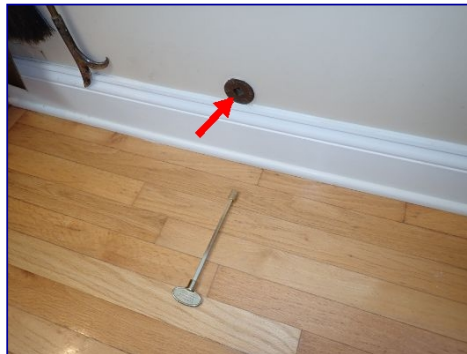
FYI: Fireplace gas shutoff valve. Family room.
