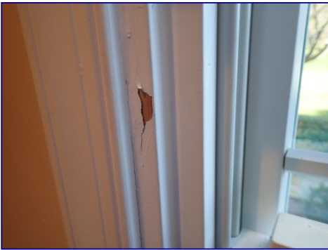
Paint failed. Office window frame.
