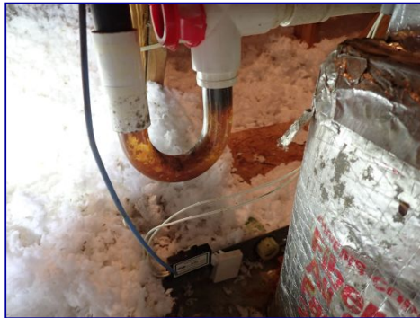
Trap dirty. Condensate drain line. Attic.
