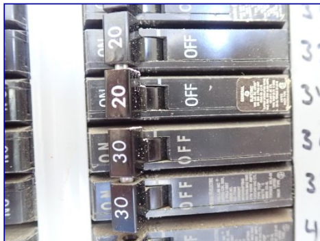
Breaker undersized. A/C minimum 36.6A, 20A or 30A installed.
