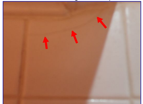
Tile cracked, not loose. Basement bathroom.
