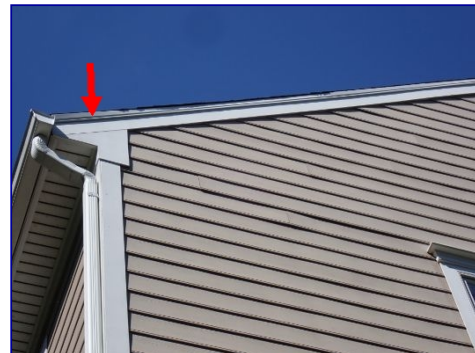
Trim or trim wrap loose. SE side rear rake.
