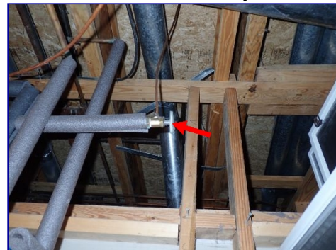
FYI: Refrigerator water line shutoff valve. Utility closet.
