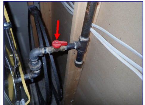
FYI: Furnace gas shutoff valve. Utility closet.
