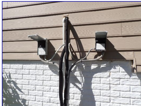
FYI: Heat pump service disconnects. SE side.
