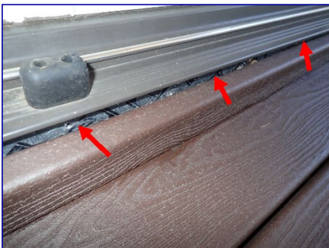
Sealant missing. Door threshold. Rear.
