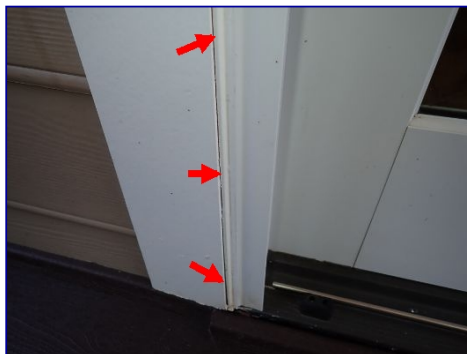
Caulk failed. Rear door frame.
