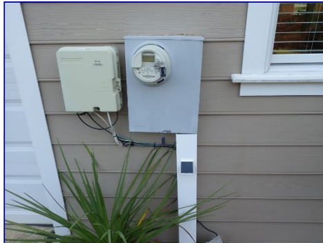
Meter settled. Sealant failed. NW side.
