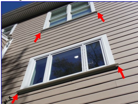
Trim misaligned. Window sills at siding.
