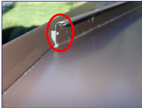
Metal standing seams single-locked. Sealant missing on top ends.
