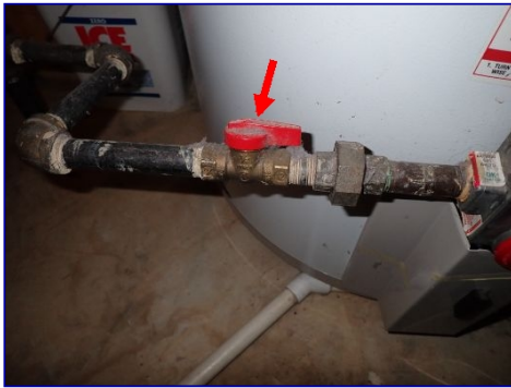
FYI: Water heater gas shutoff valve. Utility closet.
