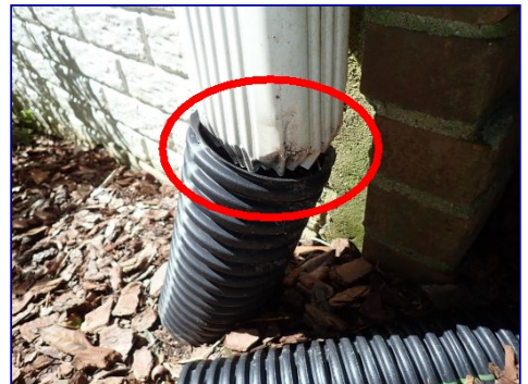
Downspout extension adapter missing. Front east corner.
