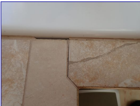
Caulk missing. Grout cracked. Bathtub perimeter.
