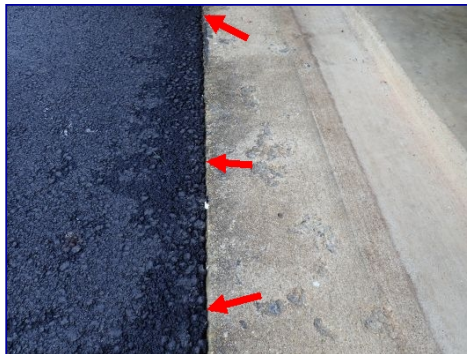
Sealant missing. Driveway at garage.
