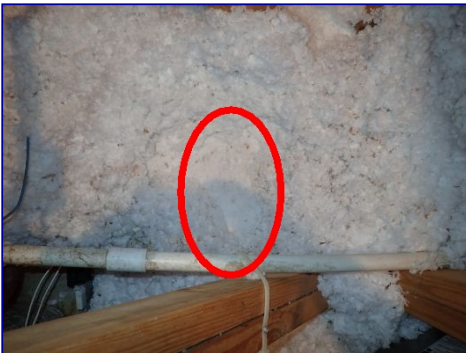
Insulation compressed. Footstep.
