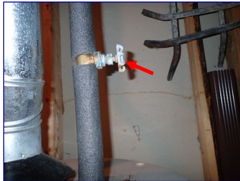
FYI: Water heater cold water shutoff valve. Utility closet.
