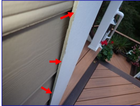
Paint missing. Cut edges.
