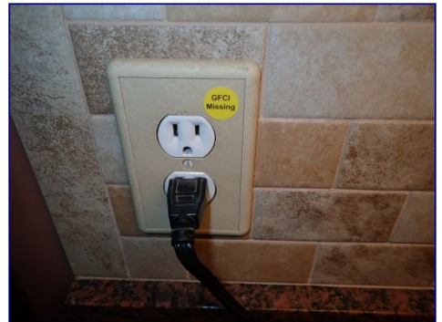
GFCI protection missing. Kitchen countertop next to refrigerator.
