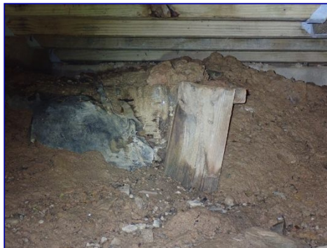
Wood in contact with soil. Under rear deck.
