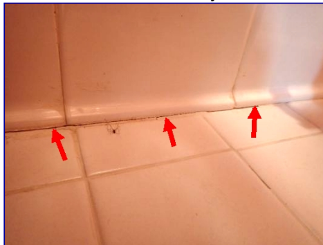
Caulk missing. Floor perimeter. Basement bathroom.
