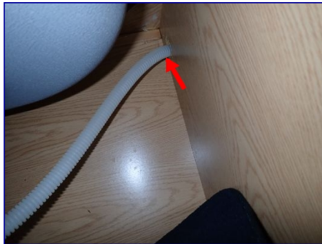
Dishwasher drain high loop low. Under kitchen sink.
