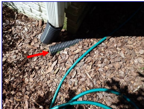
Downspout extension discharges at foundation. Perforated pipe installed. Front east corner.
