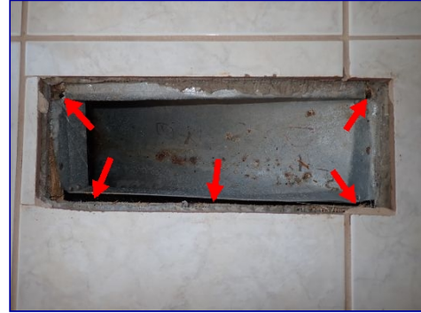
Sealant missing around floor register boxes.
