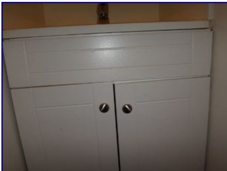
Cabinet misaligned. Doors misaligned. Half bathroom.
