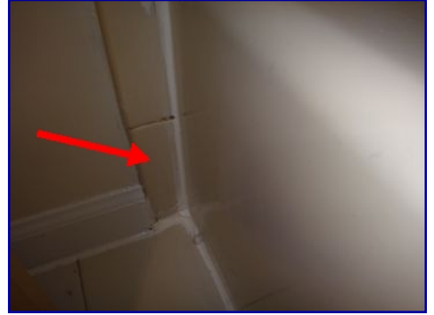
Tile loose. Upstairs bathroom.
