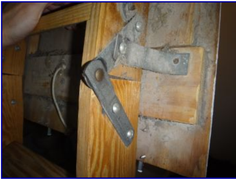
Hardware loose. Pull-down stairs.
