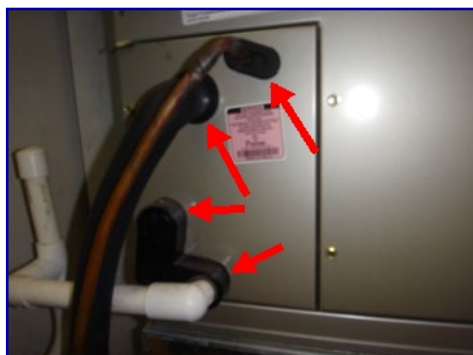
Sealant missing. Cabinet penetrations.
