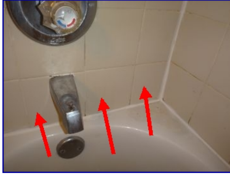
Tiles loose. Upstairs bathroom.
