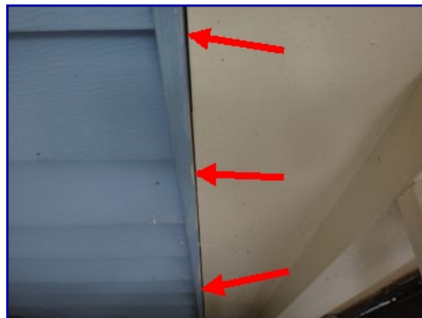
Caulk missing. Siding at trim.
