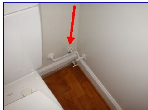
FYI: Exterior hose bib shutoff valve. Half bathroom.
