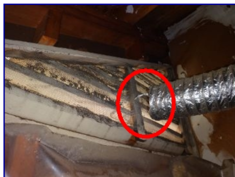
Exhaust vents to attic.
