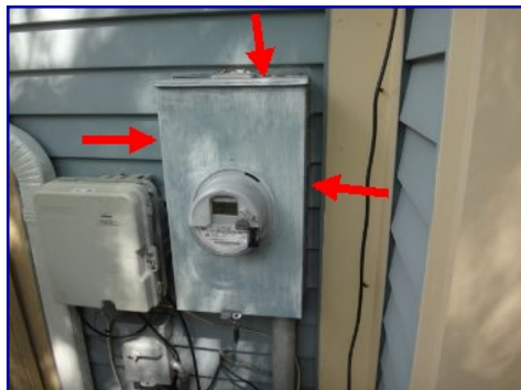
Caulk failed. Electric meter perimeter.
