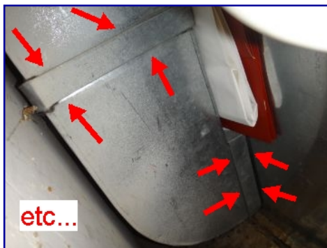
Sealant missing. All joints and seams.
