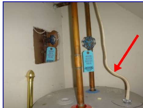
Service disconnect missing. Water heater.
