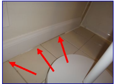
Caulk missing. Floor perimeter. Upstairs bathroom.
