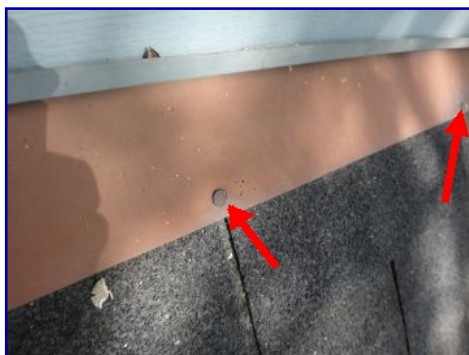
Rust visible. Sealant missing. Porch roofing.
