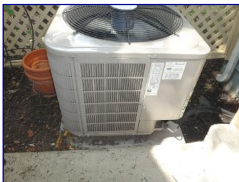
Condenser out-of-plumb. Base low.
