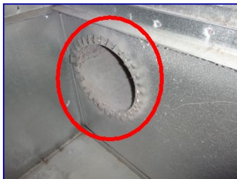
Sealant missing. Return air duct.
