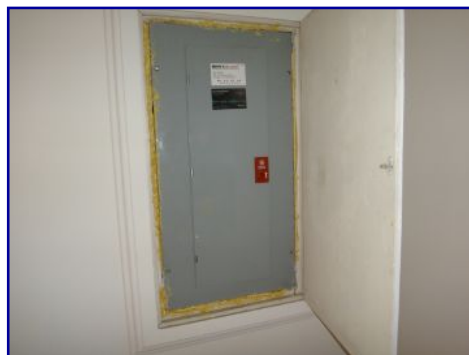
Repair visible. Electric panel perimeter.
