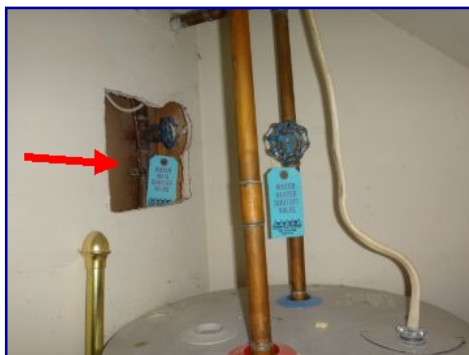
Hole in wall. Water main.
