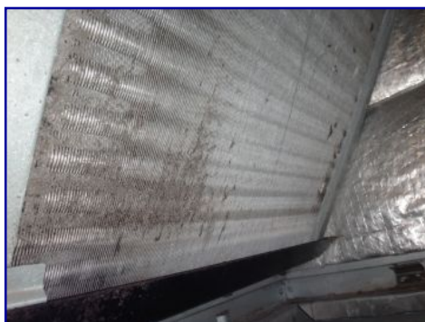
Evaporator coil dirty. Inside cabinet.
