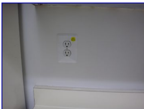
GFCI protection missing. Kitchen.
