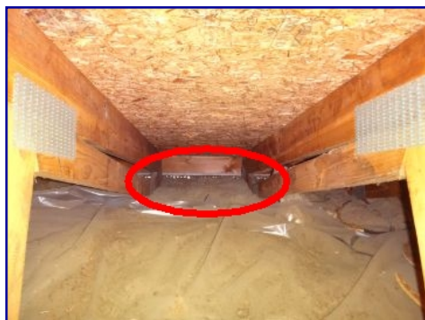
Insulation baffles missing.
