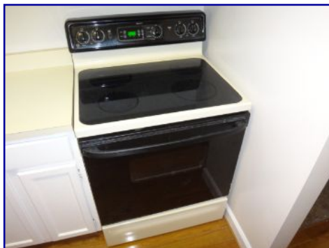
Anti-tip bracket missing.
