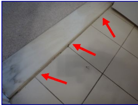
Caulk missing. Floor perimeter. Upstairs bathroom.
