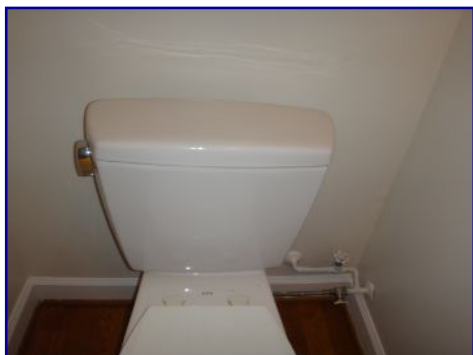
Toilet tank loose. Half bathroom.
