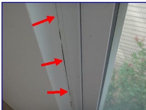
Caulk failed. Window frame. North bedroom.
