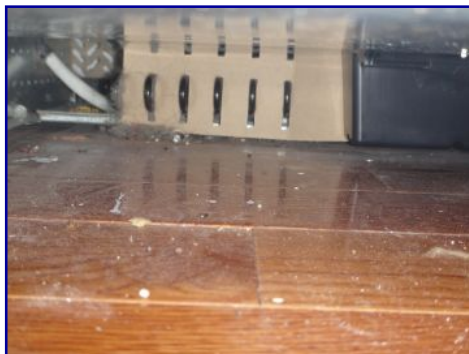
Coils dirty. Refrigerator bottom rear.
