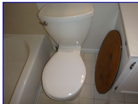
Toilet loose at floor anchor bolts. Upstairs bathroom.
