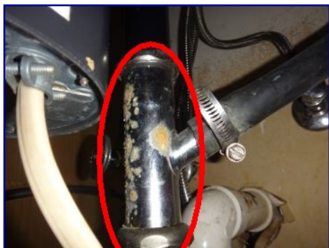
Corrosion visible. Kitchen.
