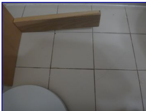
Tiles loose. Upstairs bathroom.
