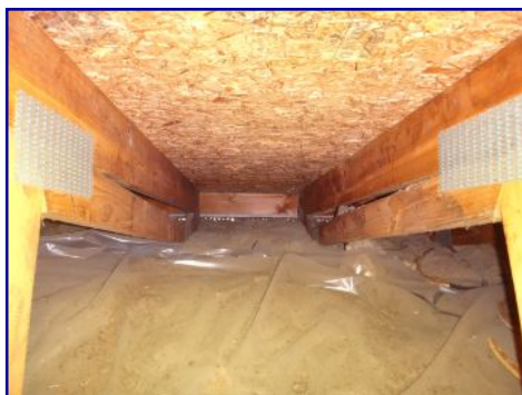
Insulation low. Moisture barrier on wrong side.
