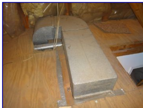
Sealant missing. Joints and seams. Insulation missing. Attic.
