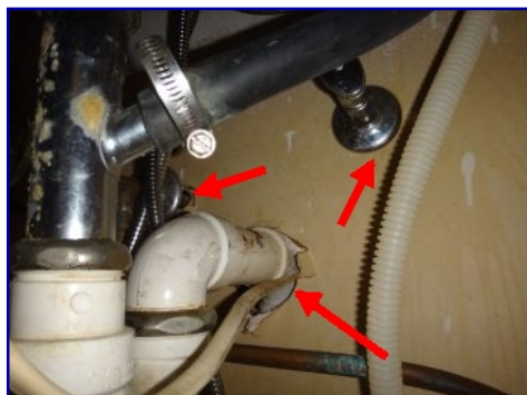
Holes in wall. Plumbing penetrations under sinks.
