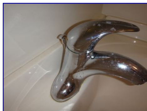
Drain stopper inoperable. Half bathroom.
