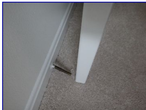
Door stop damaged. North bedroom.
