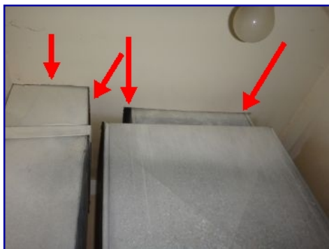
Hole in ceiling. Duct penetrations. Air handler closet.
