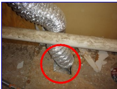
Excessive duct length. Duct compressed. Upstairs bathroom.
