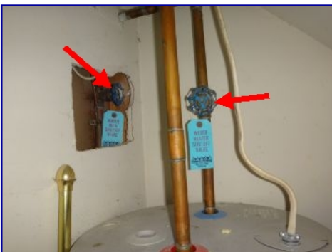
FYI: Main and water heater water shutoff valves.
