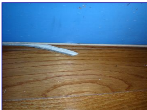
Weatherstripping damaged. Door bottom. Front door.
