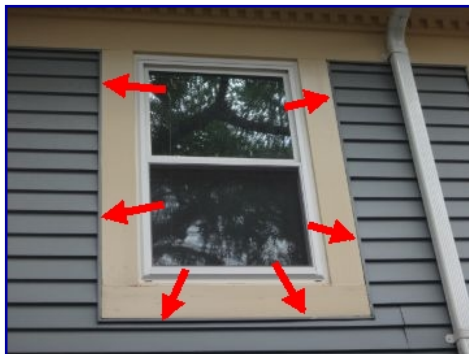
Caulk missing. Siding at trim.
