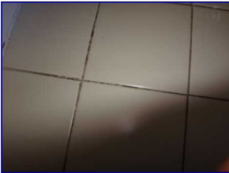
Grout stained. Sealant missing. Upstairs bathroom.
