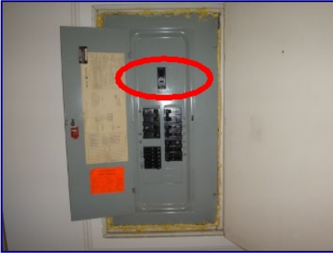
FYI: Main disconnect in panel. Panel located in living room.
