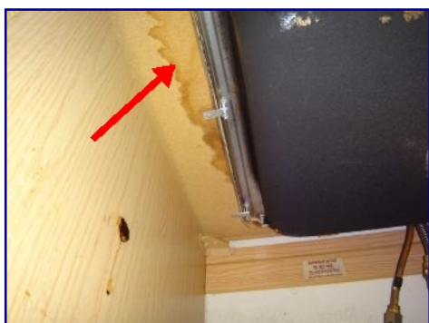
Water stain. Under kitchen sink, left side.
