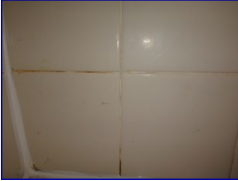
Grout stained. Sealant missing. Upstairs bathroom.
