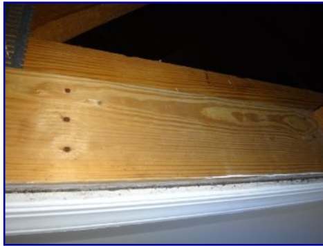
Fasteners wrong type. Pull-down stairs frame.
