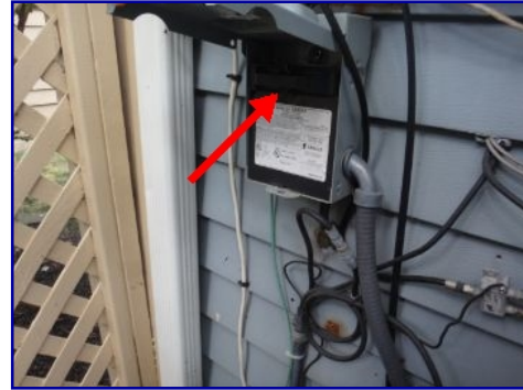
FYI: Heat pump service disconnect.
