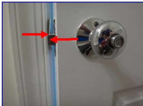
Strike plate misaligned. Upstairs bathroom.
