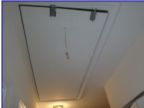
Seal missing. Pull-down stairs.
