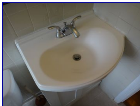
Sink loose. Caulk failed. Bathroom.
