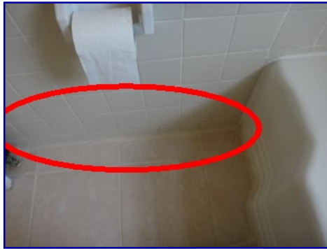
Tile loose. Bathroom.
