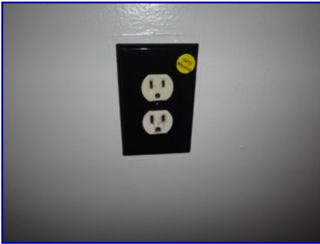
GFCI protection missing. Kitchen countertops.
