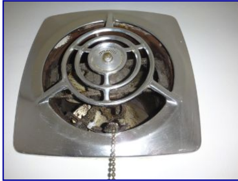
Fan dirty. Grease buildup.
