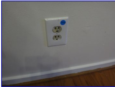
Receptacles worn. Numerous receptacles. Light blue dots.
