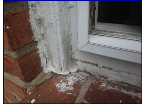
Paint failing. Caulk failed. All window frames.
