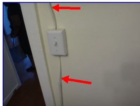
Wire subject to damage. Conduit loose. Dining room.
