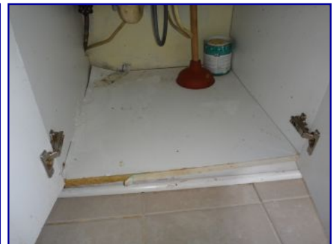
Evidence of pests. Shelf damaged. Kitchen.
