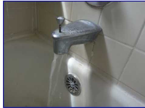
Diverter leaking.
