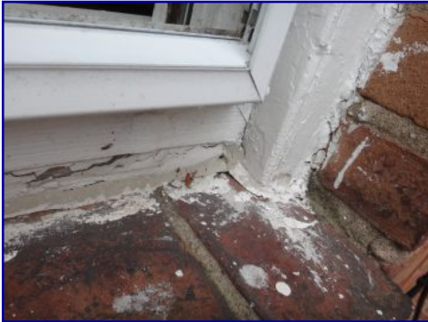
Paint failing. Caulk failed. All window frames.
