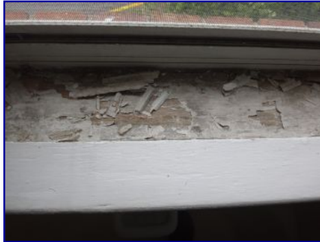
Paint failing. Window sills.
