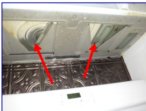
Grease filters missing.
