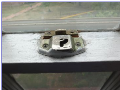
Locks damaged. Numerous windows.
