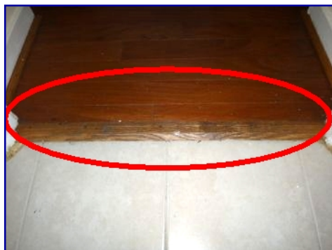
Flooring damaged. Threshold loose. Kitchen.
