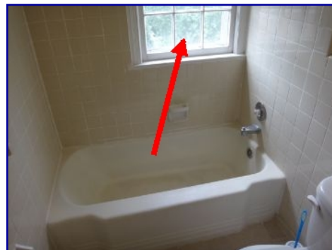
Safety glazing not visible. Bathroom.
