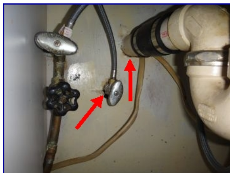
Holes in wall. Plumbing penetrations under sinks.
