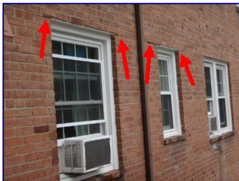
Lintels rusted. Mortar cracked.
