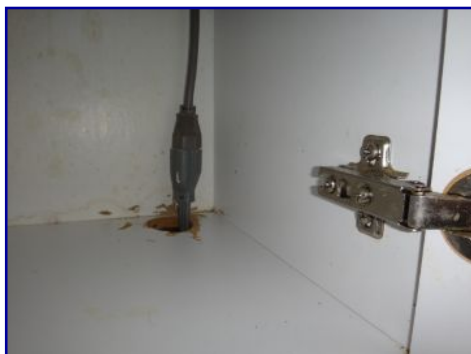
Extension cord wiring. Microwave.
