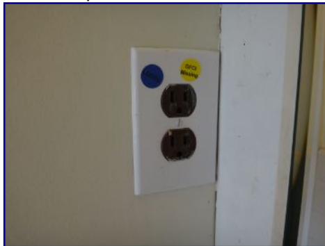
GFCI protection missing. Receptacle loose. Bathroom.
