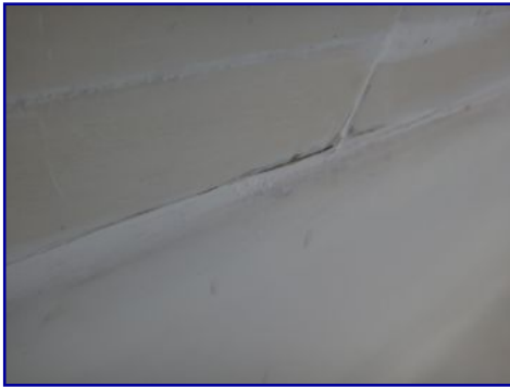
Caulk failed. Bathtub perimeter.
