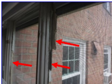
Glazing compound failed. Paint failing. All windows.
